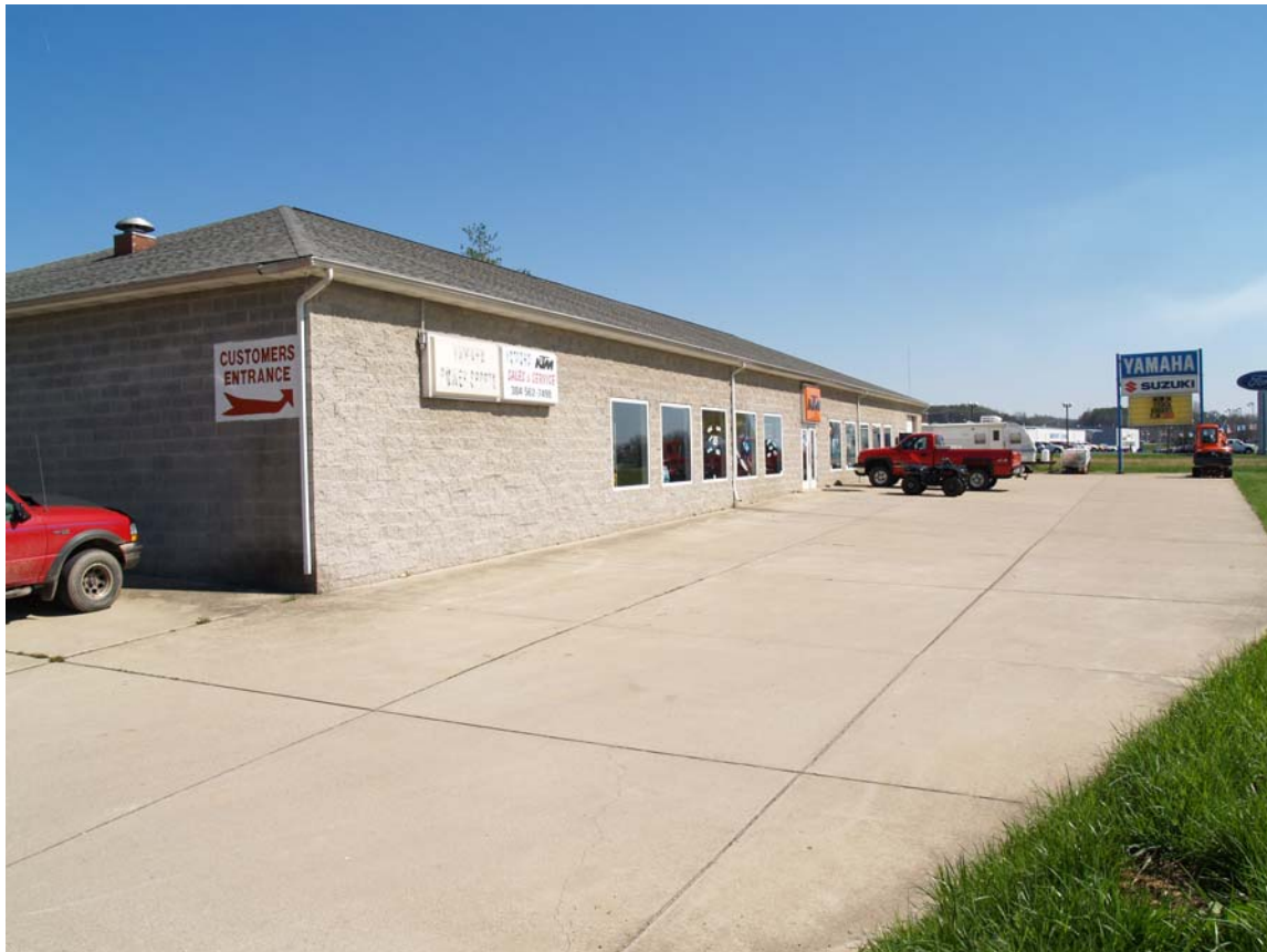
Front view of building from south side, (I-64, interstate side of building) (04/17/09)
