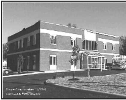
A & L Office Building, Cow Creek Rd. & SR 34
