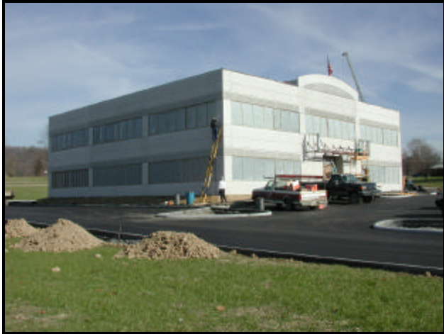
Charter's new facility takes shape (12/04/00)
