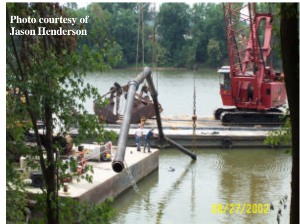
A major undertaking—placement of sewer line on the bottom of the Kanawha River. The new line will serve the Putnam Business Park.
