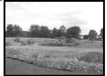
Charter site work underway
