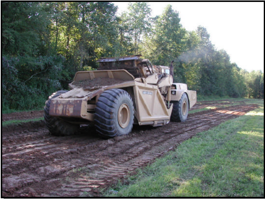
A pan scraper removes the topsoil on the ridge at the south side of the existing wetlands at Putnam Business Park in preparation for Phase II archeological work at the site. (9/6/01)
